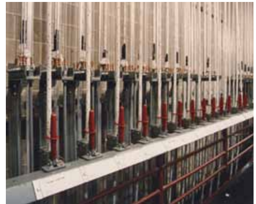
Typical Underhung Counterweight System
